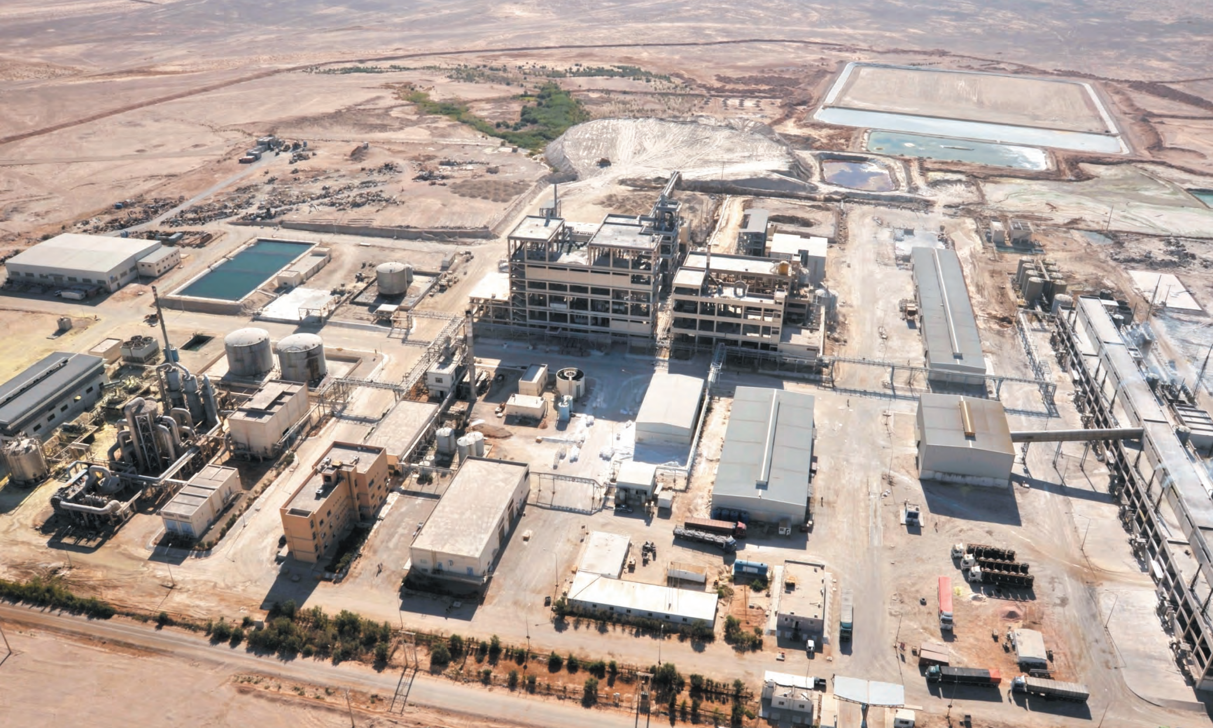
Jordan Abyad Chemical Complex
