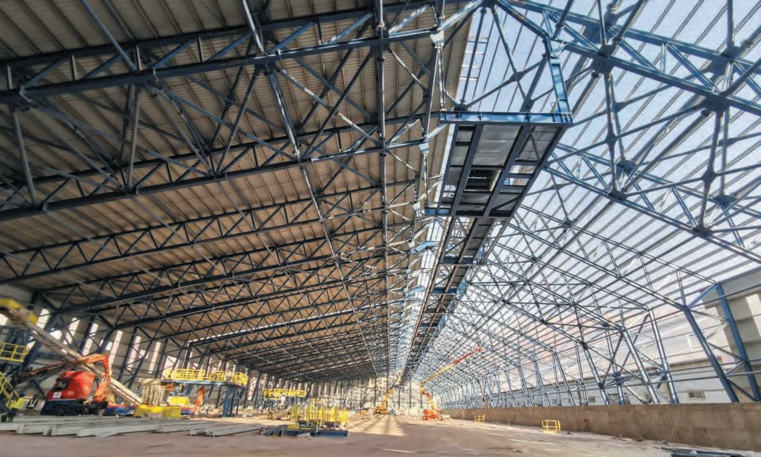
Potash Management New Hangar
