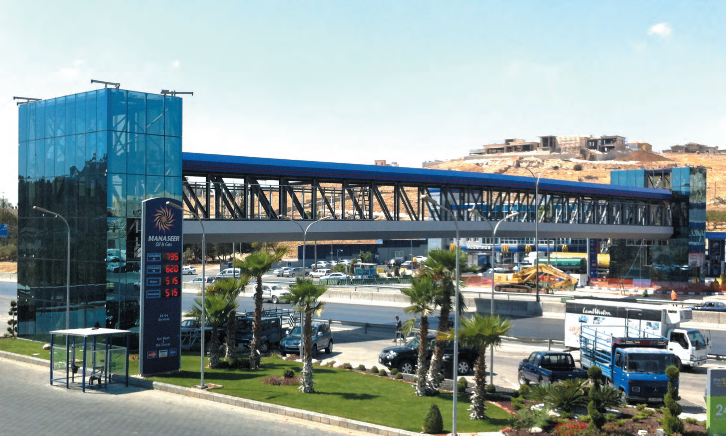
Airport Highway Pedestrian Bridge
